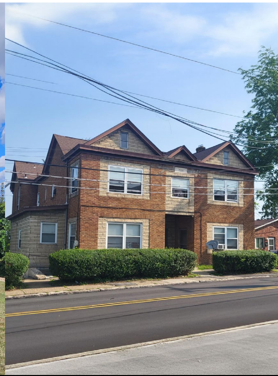
2769 CHURCHVIEW AVE 10 UNITS
