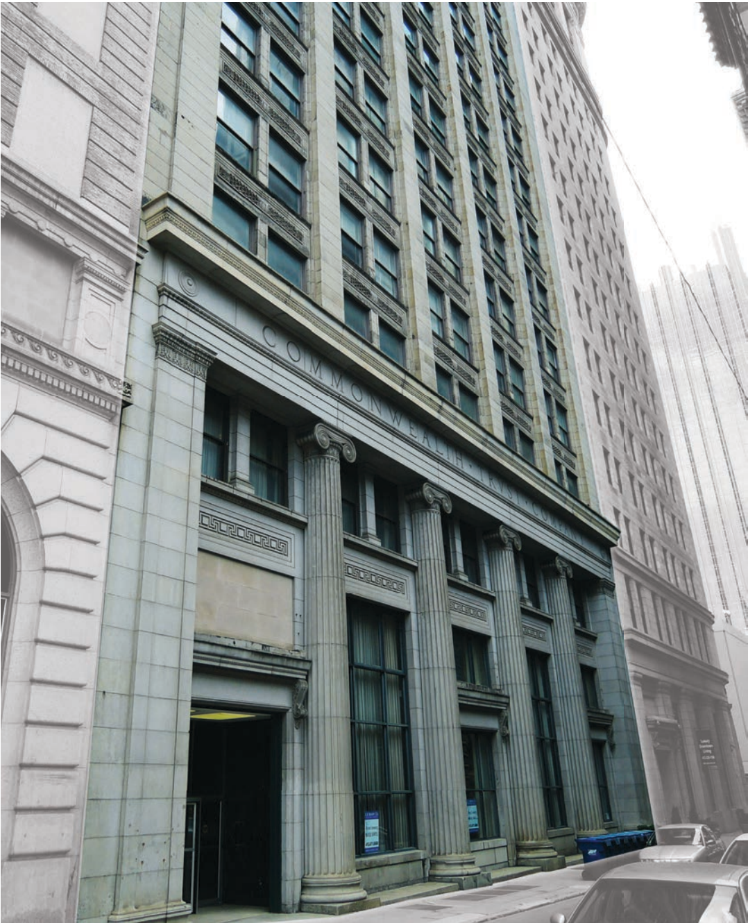
Current Lobby Condition - Active Staging Area
